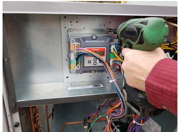
Figure 7 – Mount Controller Assembly in Unit Control Box
